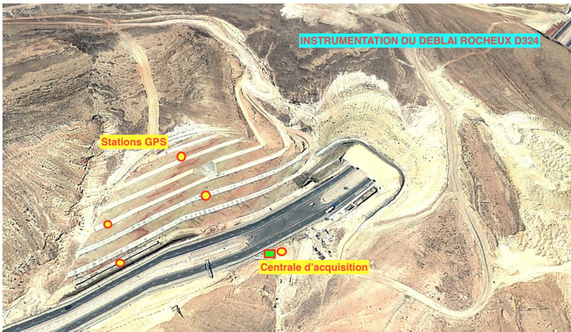
Figure 6. Instrumentation implemented on D324.
