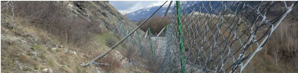
Figure 5. Filets pare-blocs, (Cerema 2021).
