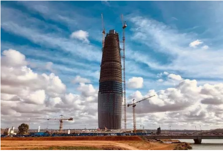
(a) Mohammed VI Tower - Exterior View
